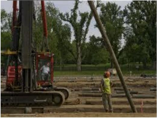
All temporary casings are to be extracted immediately after completion of concreting. A vibro-Hammer will be used to extract the casing.
