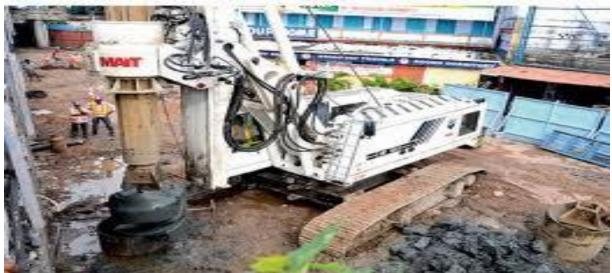
This Work Method Statement outlines the method of which the bored piling works are installed for the project.
